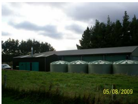
Exterior view of new LCT facility
